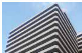
S8 Sumitomo Electric Hardmetal (Thailand) Ltd.
